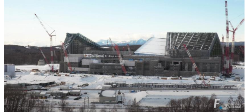
F. Village construction in progress (December 2021)
