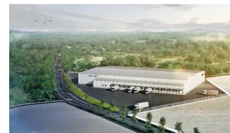
LOGITRES Chiba (tentative Name) logistics facility
