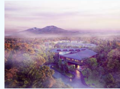
OST Residence Karuizawa
