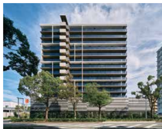
Le JADE Kakegawa Ekimae (Kakegawa City, Shizuoka Prefecture) (83 units in total) [Condominium]
