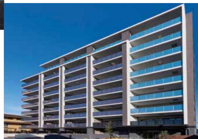
Grand Clare Ichinomiya (Ichinomiya City, Aichi Prefecture) (41 units in total) [Condominium]
