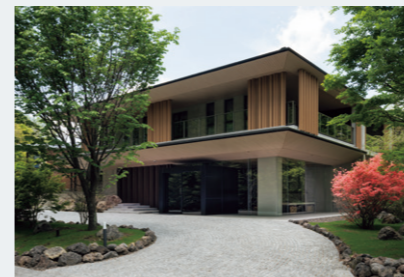
OST RESIDENCE KARUIZAWA
