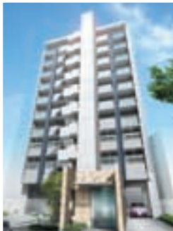
Leaf Comfort Kiyosumi-Shirakawa Situated near central Tokyo, this rental condominium complex for singles was fully occupied immediately after completion. Its success reflects sophisticated design features and superb product characteristics.
