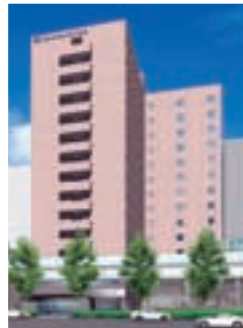
Kawasaki Ekimae PJ (business hotel) ES-CON Japan plans to build a business hotel near Kawasaki Station with retail outlets on its lower floors. Major companies have offices in this area. The project is to provide reliable income by leasing the building to a hotel management company.
