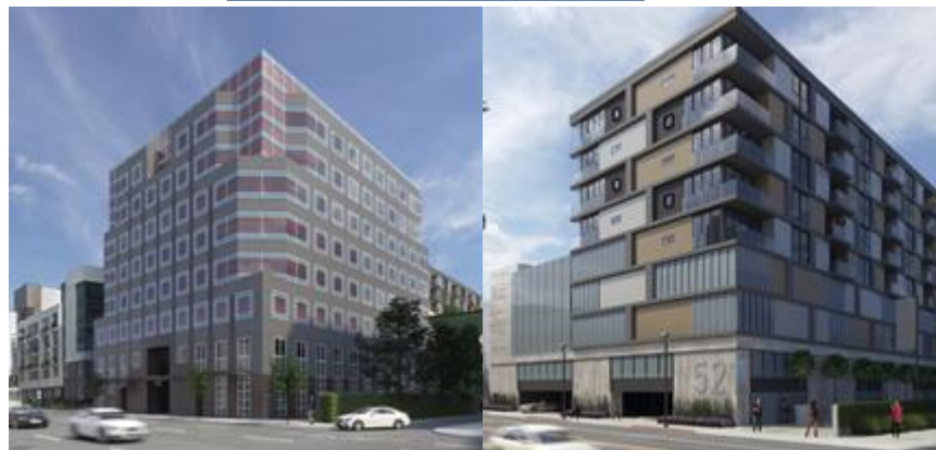
Exterior of Tower 520 N. Central
