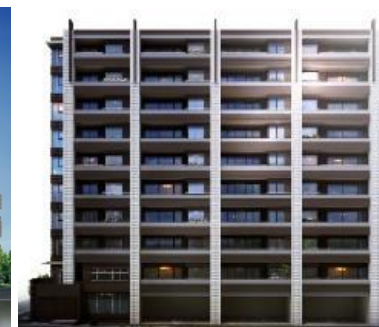
Le JADE Ikeda Masumicho (Osaka) Location: Ikeda-shi, Osaka Access: 2-minute walk from Ikeda Station on Hankyu Takarazuka Line No. of residences: 35 Occupancy date: Late May 2020
