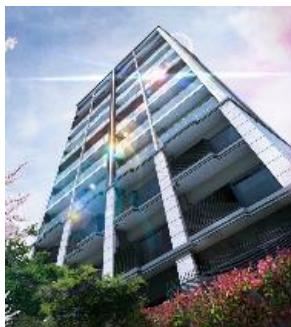
Le JADE Higashisumiyoshi Imagawa Ryokudo (Osaka) Location: Osaka-shi, Osaka Access: 4-minute walk from Tobushijomae Station on JR Kansai Main Line No. of residences: 41 (plus one management office) Occupancy date: Late February 2020
