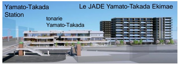
Yamato-Takada Station Le JADE Yamato-Takada Ekimae tonarie Yamato-Takada Opened in 2018 with 68 tenants as a facility with roots in the local community scaled to meet the needs of the area
