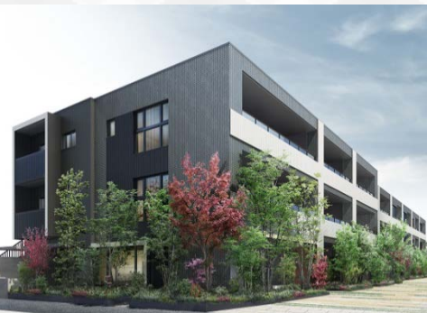
Le JADE Nakano (Metropolitan area) Location: Nakano-ku, Tokyo Access: 13 mins. walk from Nakano Station on JR Chuo/Sobu Lines 13 mins. walk from Nakano Station on Tokyo Metro Tozai Line 12 mins. walk from Higashi Nakano Station on JR Chuo/Sobu Lines 11 mins. walk from Higashi Nakano Station on Toei Oedo Line No. of residences: 25 Occupancy date: To start at end of December 2018
