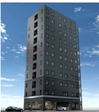
Kayabacho, Nihonbashi Opened in December 2016 102 rooms
